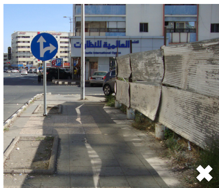
Figure 185 Temporary fencing with corrugated sheets
