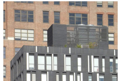
Figure 182 Example of rooftop equipment screening well-integrated into the total building design
