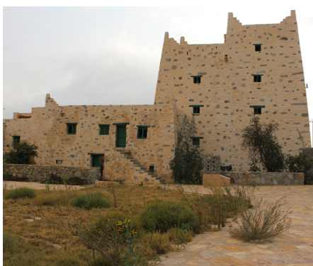
Figure 141 Heritage architectural styles of the Aseer region and typical construction materials used: natural stone, mud, clay and timber
