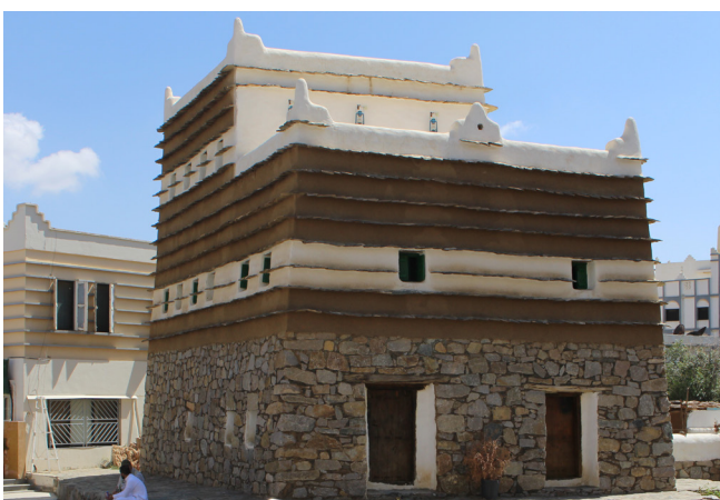
Figure 40 Example of facade treatment present in the Sarwat Mountain's vernacular architecture
