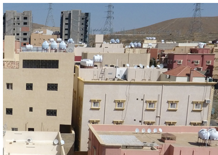
Figure 180 Example of unscreened visible rooftop equipments
