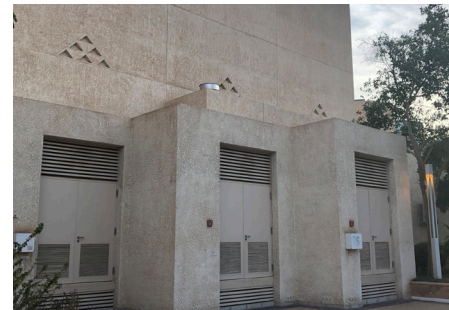
Figure 176 Example of fully screened refusal area integrated within the design of the building
