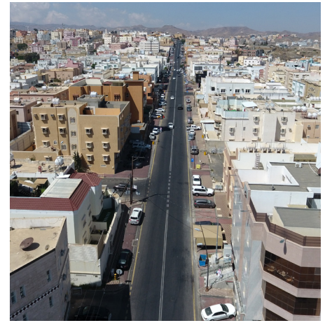
Figure 155 Uniform scale with gradual variation provides street wall and well balanced view
