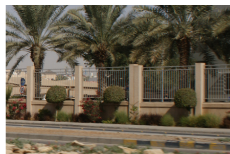
Figure 172 Fence integrated with landscape and allowing more transparency
