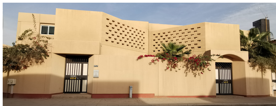
Figure 189 Example of screening elements included into the overall architectural design in terms of material, color and pattern
