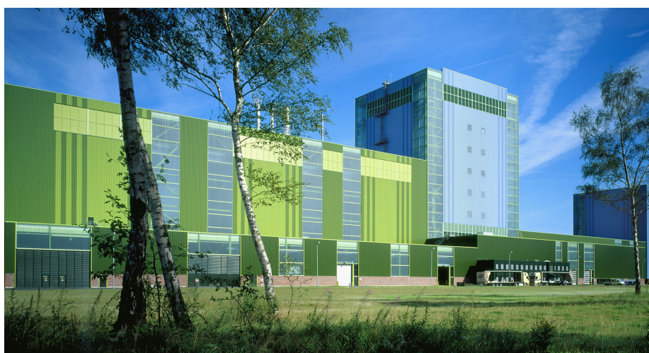
Figure 201 An example of building massing breakdown and harmonious color arrangements: The FBA 8 hot-dip galvanizing plant in Dortmund comprises three hall sections arranged in parallel with one another in accordance with a color concept by Friedrich E. v. Garnier (Credits: ThyssenKrupp Rasselstein GmbH, Andernach)
