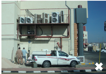
Figure 174 Example of exposed services and utilities
