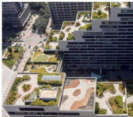
Figure 181 Green stepped terraces with furniture on roof top and appropriately screened equipments
